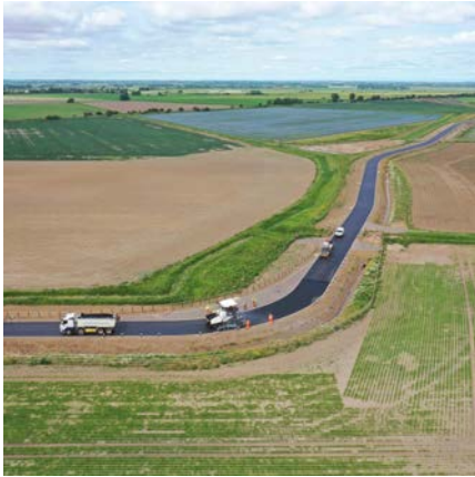
Rated Excellent Viking Link (Bicker Fen) Access Road, 2021 Lincolnshire, England
