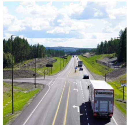
Rated Excellent Rv3/Rv25 new highway between Løten-Elverum Norway
